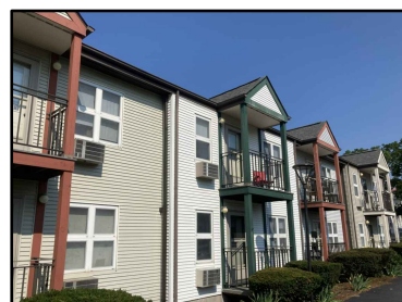
TYPICAL EXTERIOR BLDG DECK
