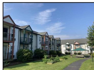
TYPICAL EXTERIOR BLDG VIEW
